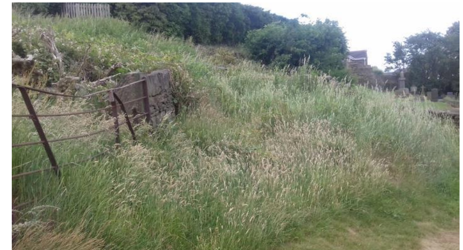
Photo 30: Route widens out, old iron field gate on right, 2 Vermont Close visible in distance, looking towards overgrown point E leading north-west 22/6/2017
