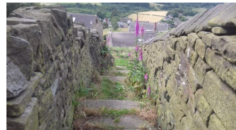
Photo 18: Looking back down flight of stone steps towards point B 22/6/2017
