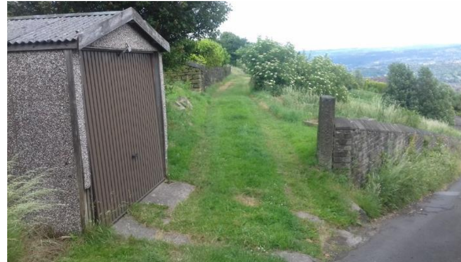
Photo 26: Point A junction of application route with Old Lane, wide grassy lane with vehicle tracks, garage of 35 High Street on left 22/6/2017
