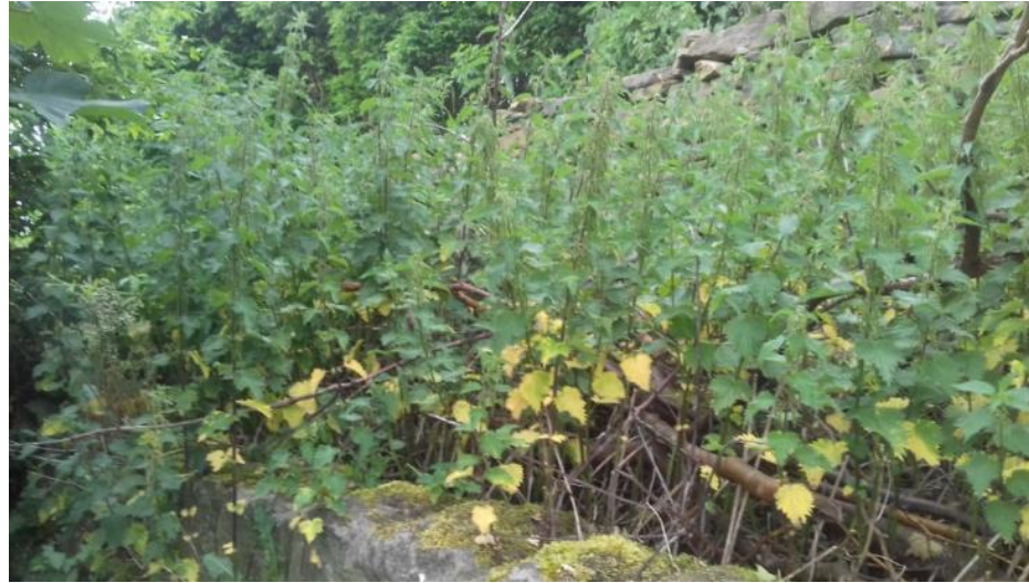
Photo 32: Narrow double walled route between point E and gate to 2 Vermont Close, overgrown, point G 22/6/2017
